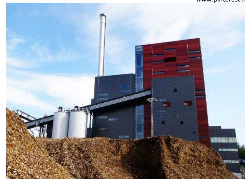
CHAUFFERIE BIOMASSE – PHOTO SUNVALOR
